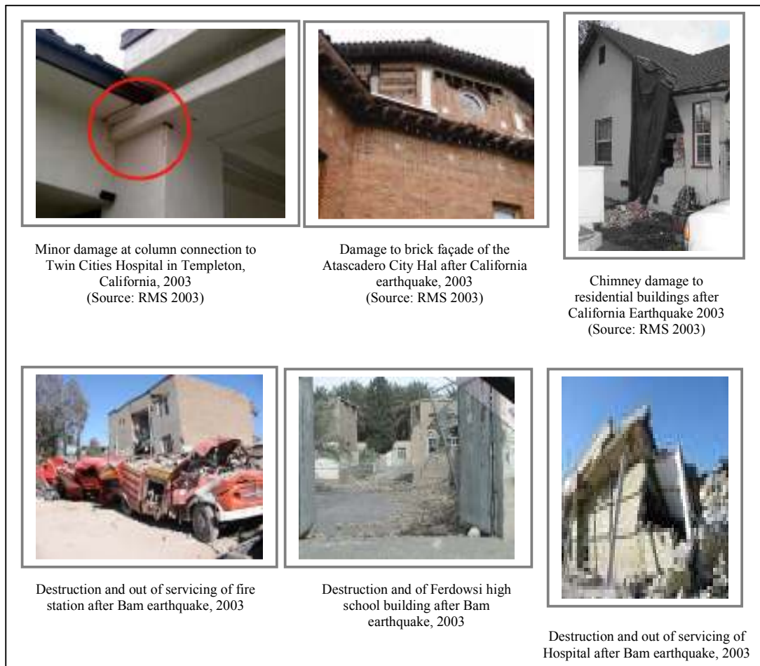
Plate 2- Comparison of California and Bam buildings destruction in the earthquakes 2003
