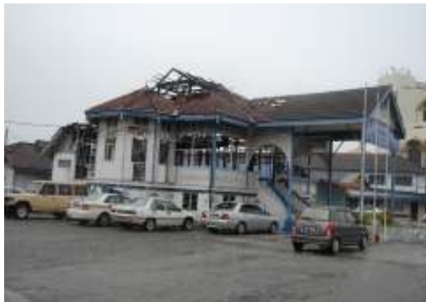
Figure 1: The 98-year old wooden building of Ipoh Volunteer Police Mess Hall was destroyed by fire on 24 July 2007.
