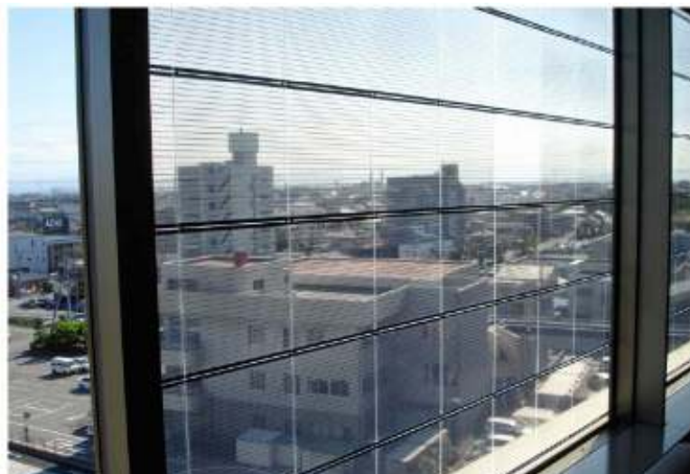
Figure 8. Building integrated see-through PV modules by Sanyo at Ohta City Hall building.
