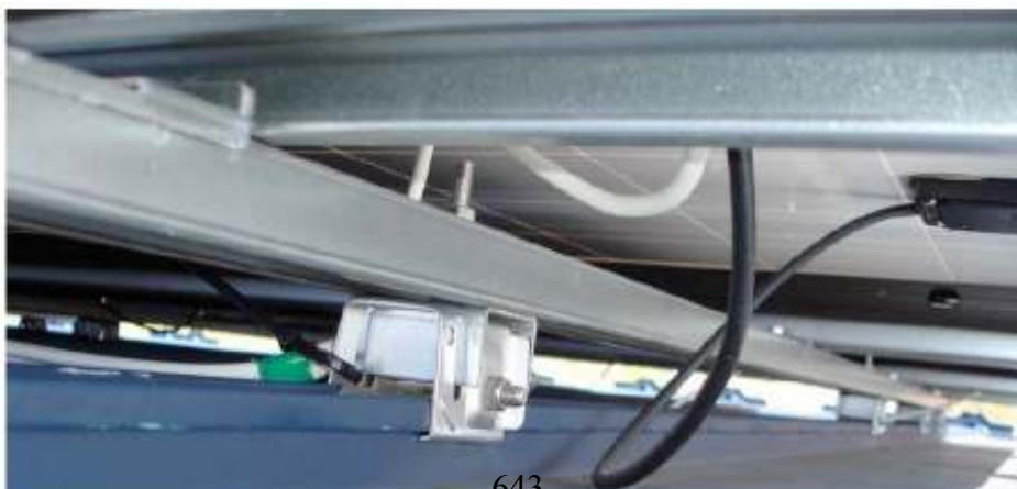
643 Figure 6. Underside of typical Japanese PV array clamp mounting on metal corrugated roof without roof penetration.
