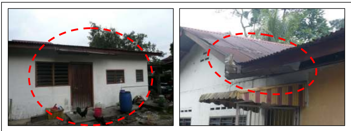
Figure 4: The back (left) and side (right) catchment of rainwater (side catchment is abandon)
