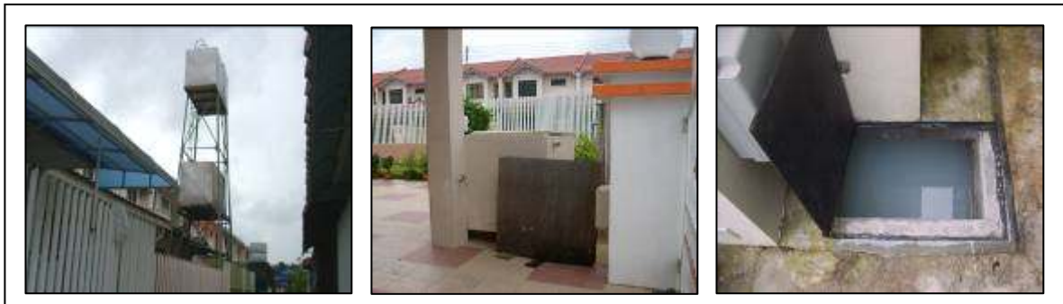
Figure 6: Backyard elevated rainwatertank (left), Frontage reinforce concrete tank (middle), and underground tank (right)
