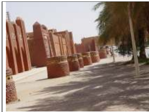
Figure 1: Foggara wells along streets in Adrar (Algeria)
