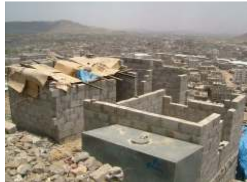
PHOTOGRAPH 4 View of the Housing Area
