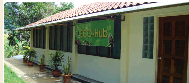
Building B11 was successfully restored by the Development Office within a month after the Eco USM Team was formed at the Ecosystem, Landscape and Heritage Workshop. Kudos to the Development Office on a job well done.
