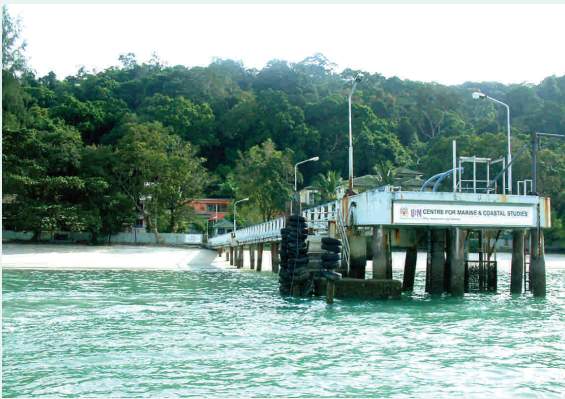
The CEMACS jetty.
