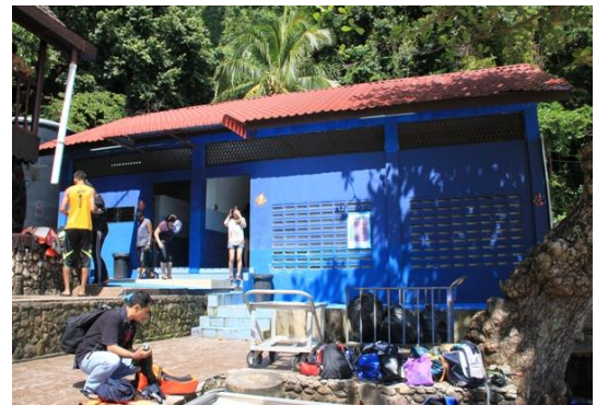
Figure 1.3 (d) Toilets and changing rooms provided for the visitors
