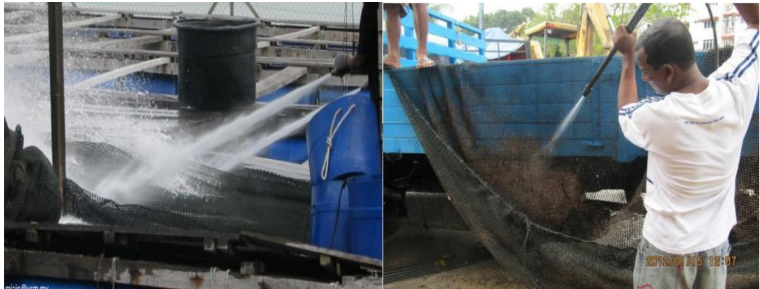
Figure 2.8: The mechanical cleaning method to control biofouling.
