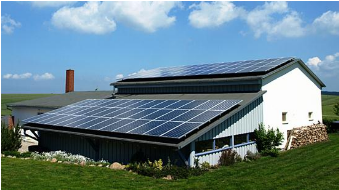
Figure 1.6: Example of Solar Panel on the Roof
