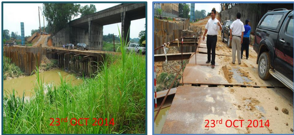
Plate 1.1 Temporary bridge at Sungai Damansara, Selangor
