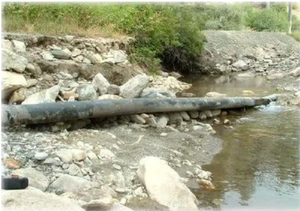
Figure 1.6 Exposed oil pipeline on Beaver Creek near Helena (Boyd et al., 2013).
