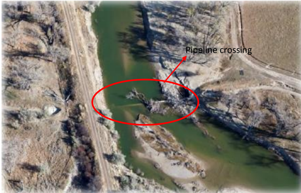
Figure 1.5 2011 flood scoured the river bed, exposing the irrigation inverted siphon on the Musselshell River (Boyd et al., 2013).
