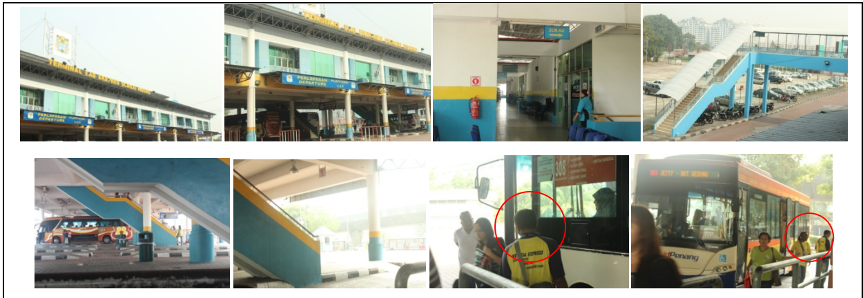
Figure 4: Views of Sungai Nibong Terminal
