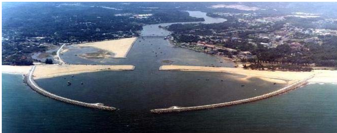
Figure 1: Breakwaters at Merang river mouth.
