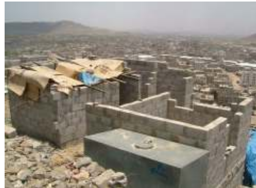
PHOTOGRAPH 4 View of the Housing Area
