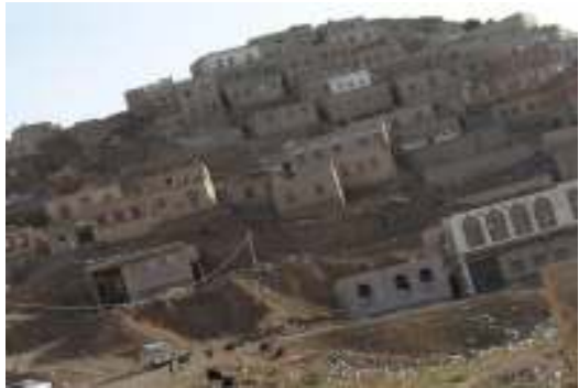
PHOTOGRAPH 1 View of Land Erosion
