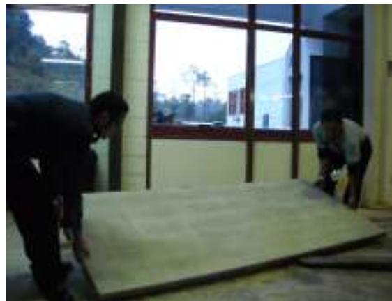
Figure 4: Two workers lifting a 2.4 m PSSDB floor panel
