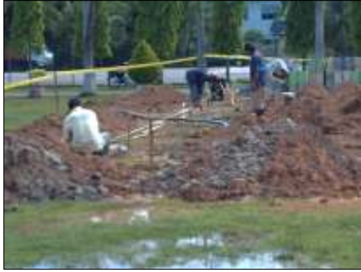
Figure 8(a). Construction of footing
