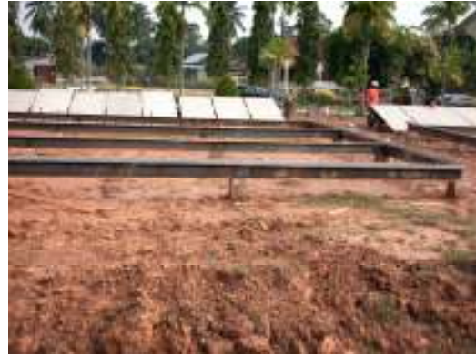
Figure 8(b). Erection of floor panel
