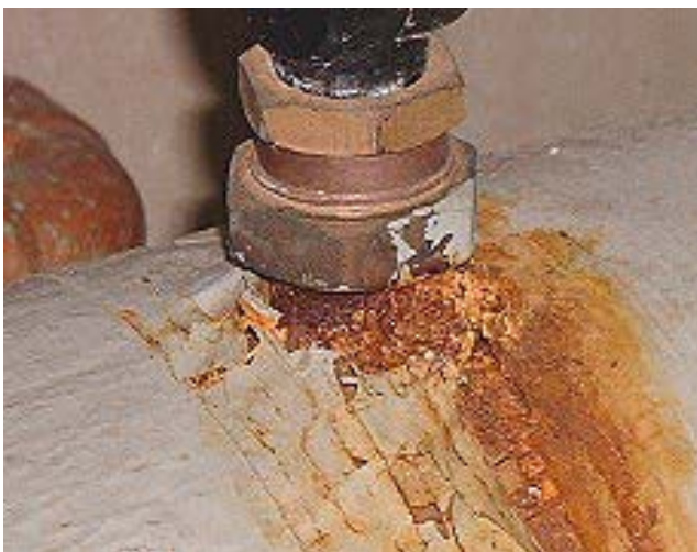
Figure 3 - Photograph showing corrosion around the copper and steel tubing in a water heater
