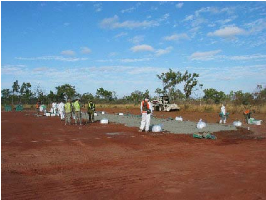
Figure 2.2: Spreading Fibres over the surface (Joint Rapid Airfield Construction, 2007)
