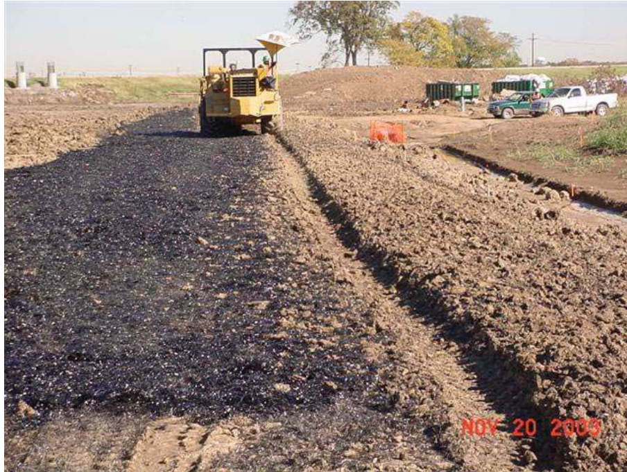
Figure 2.7: Mixing fibres with soil on the President George Bush Turnpike Project (Gregory, 2006)
