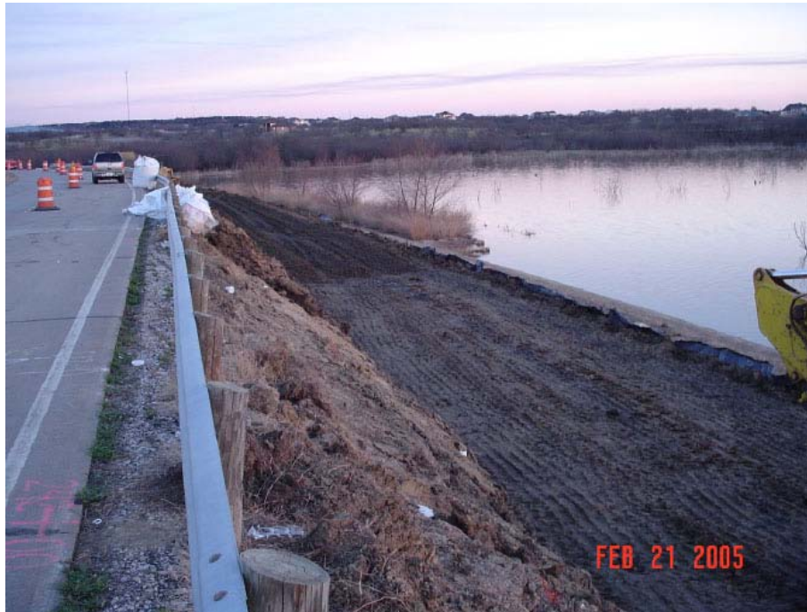
Figure 2.6: Fibre reinforced soil Embankment Construction- Lake Ridge Parkway (Gregory, 2006)
