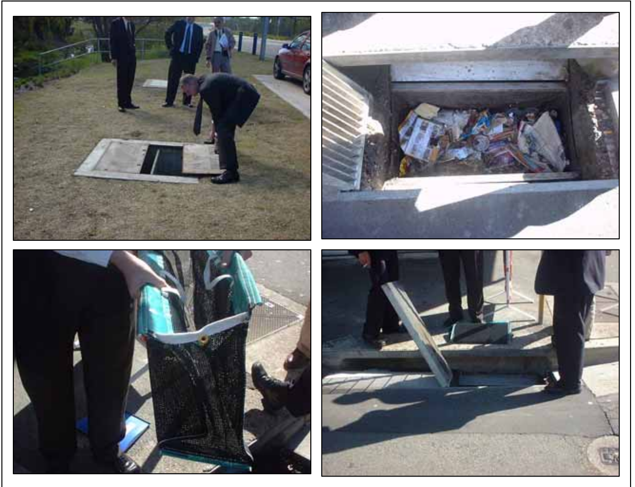
Figure 2.3: Gross Pollutant Trap (After DID Malaysia)
