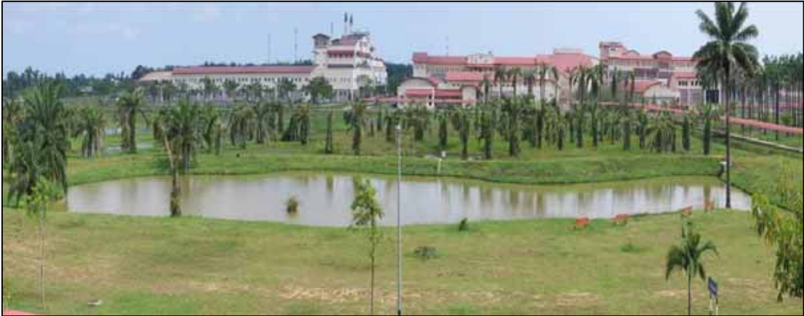
Figure 2.12: View of Wet Pond
